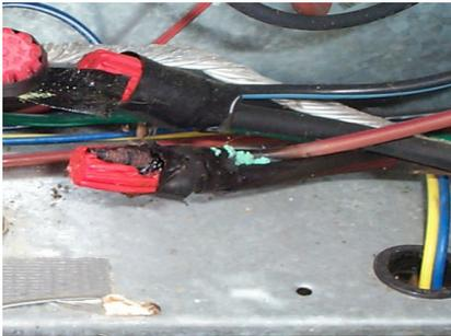
Qualified technicians should check the power connections for signs of problems or looseness. Common issues arise from off season moisture, physical and rodent damage, or corrosion.
