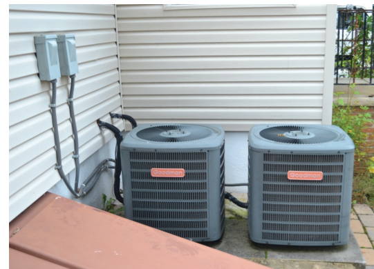
Two condensing units installed outside, but on a wall near the two furnaces in the basement
