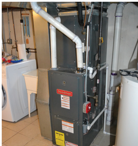
A typical forced-air furnace using gas heat and a cooling coil close-coupled to the top of the furnace
