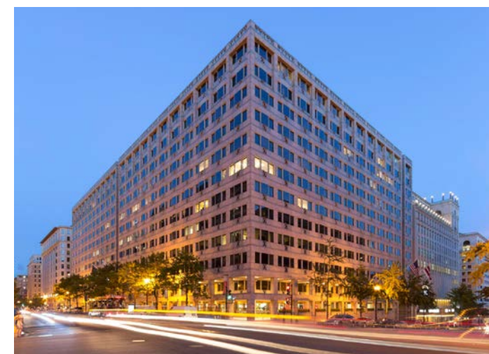
Columbia Square, Washington, LEED gold certificate
