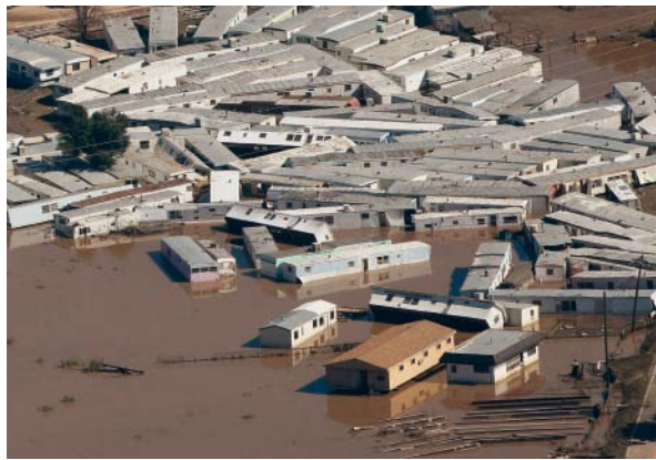
Portable buildings piled up by flood waters.
