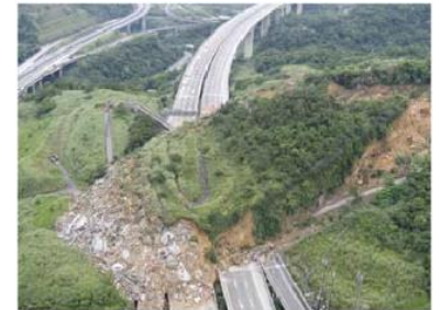
Source: Huge hillside collapses, covers Formosa Freeway
