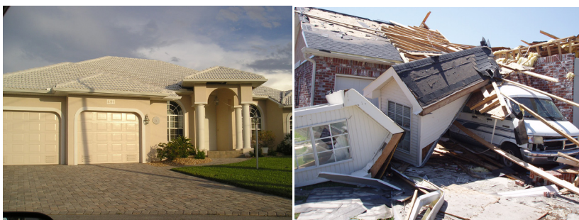
A new home in Punta Gorda, FL, (left), sustained no visible damage despite experiencing wind speeds approaching 150 mph during Hurricane Charley in 2004, while new construction near Slidell, LA, (right) did not fare as well in lower wind speeds during Katrina. A lack of statewide building codes in Louisiana and Mississippi contributed to the severity of wind damage seen after Katrina.
