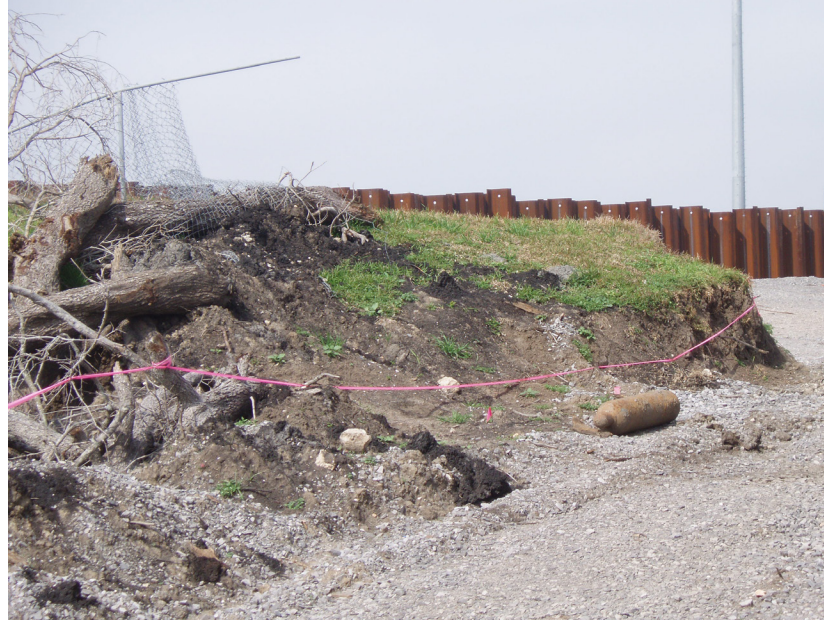
A section of damaged and eroded levee along the 17th Street Canal in New Orleans.
