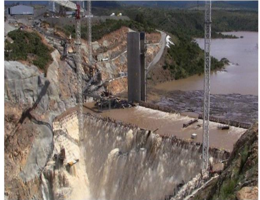
Source: floodwaters spilled over the new Cotter Dam wall
