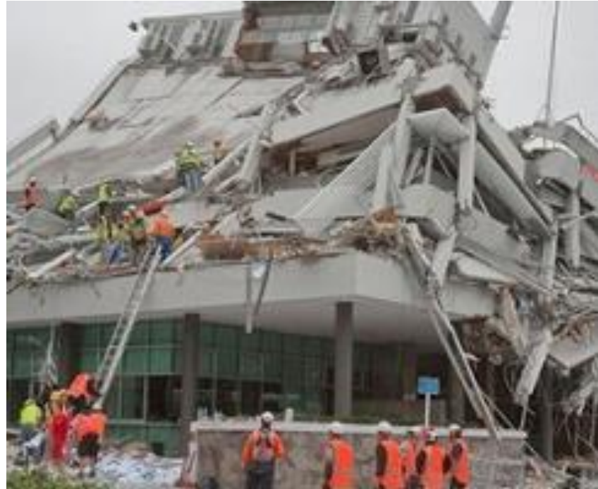
The PGC building after the February 22, 2011, earthquake
