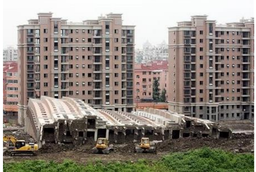
Source: Building collapse in Shanghai, China(2009)
