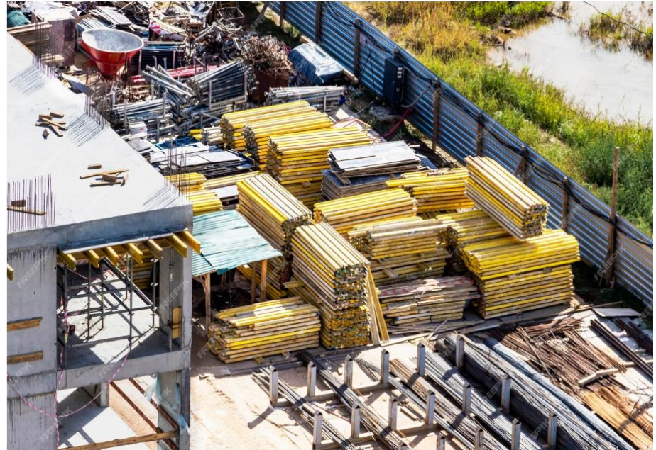
Building Material storage at the construction site
