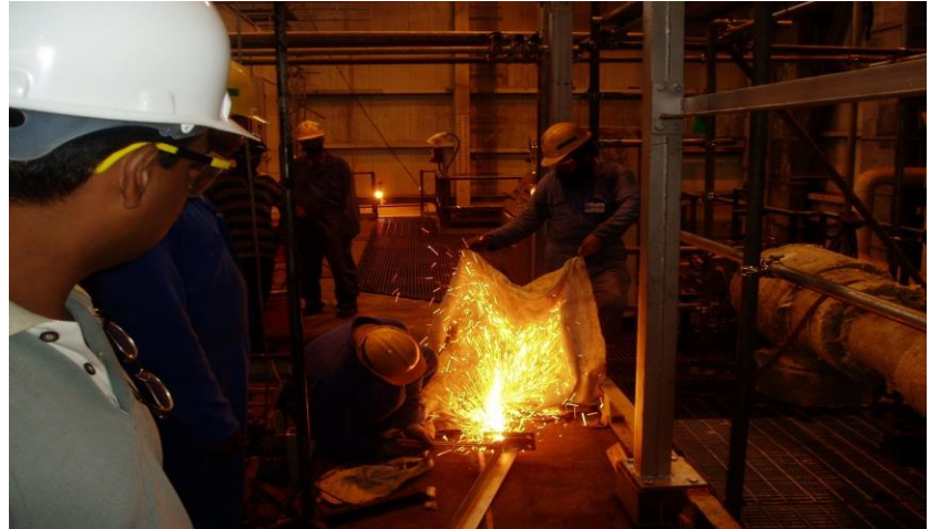
Source: Hot Works during construction
