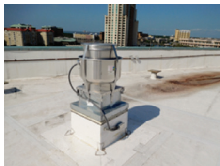
Ventilation system secured to roof
