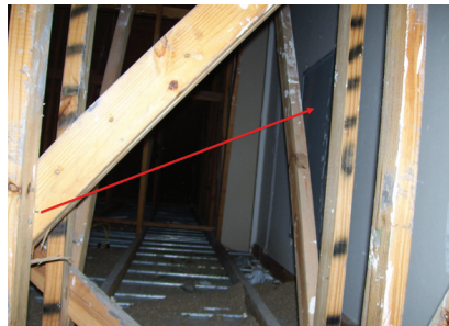
Allowed self-closing door with automatic latch in the draftstop wall of an attic.
