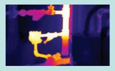
A properly operating steam trap Not all hot spots indicate a problem. This image shows a steam trap that is operating properly. Faulty steam traps waste energy; infrared thermography is an invaluable tool for readily detecting them so they can be repaired.
